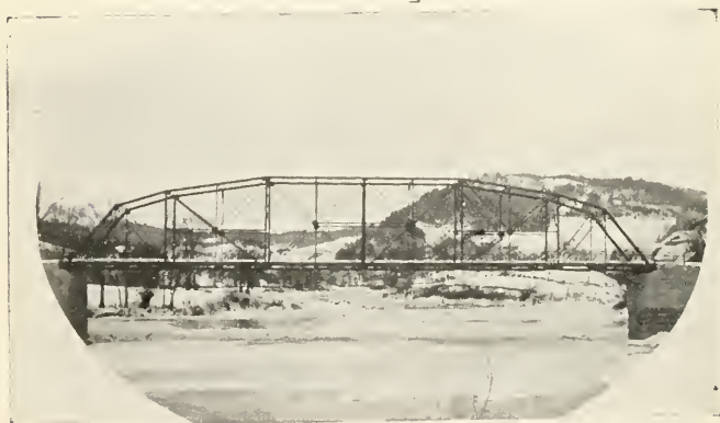
NEW IRON BRIDGE, SOUTH ROYALTON, 1903.
